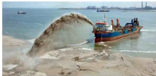
Dredging ship to prepare the barrier site and fill the cylinder (Van Oord ship)
